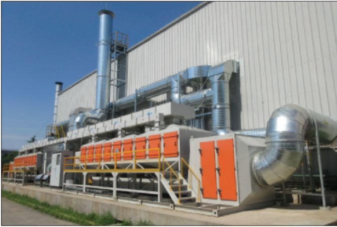
Controls to improve indoor air quality Shanghai Plant: Fresh air ventilation system
