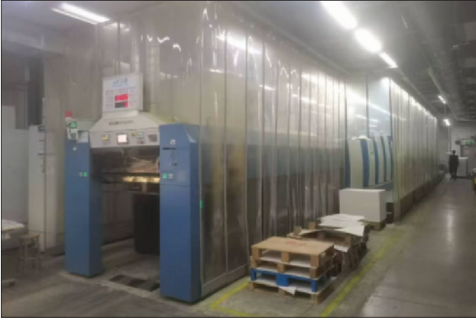
Controls to reduce employees' noise exposure Chengdu plant: engineering methods
