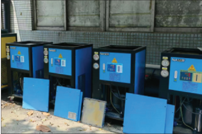
Liaobu plant (Zhuyuan): upgrade decentralized chillers to centralized chillers
