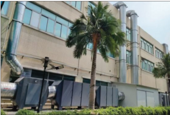
Liaobu plant (site 1&2): Exhaust gas collection and purification facilities
