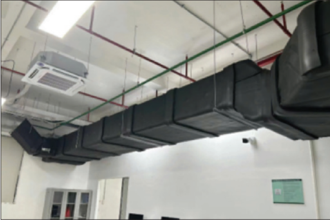
Foam plate at Bac Ninh plant to cover the air emission duct
