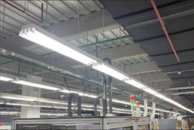
BacNinh LED lighting
